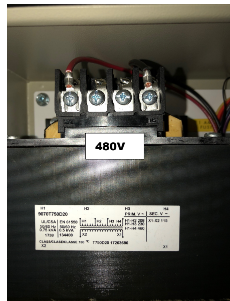
480V 3PH ONLY MODELS TRANSFORMER PRIMARY WIRING
