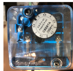
LOW PRESSURE GAS SWITCH
