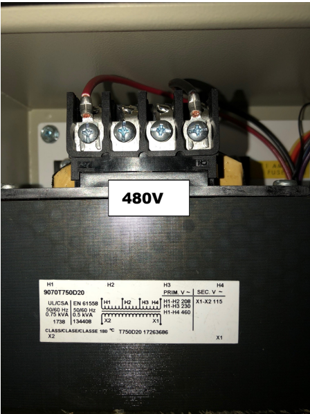
480V 3PH ONLY MODELS TRANSFORMER PRIMARY WIRING
