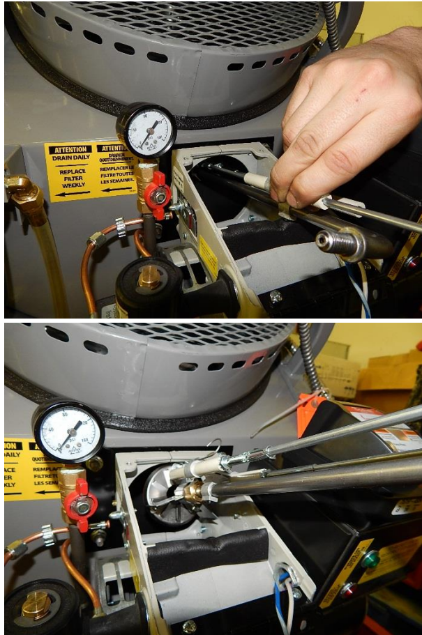
Figure 3: Assembly being pulled from blast tube
