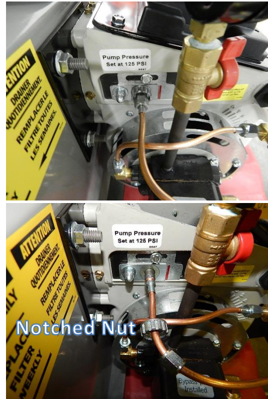
Figure 2: Copper fuel line location
